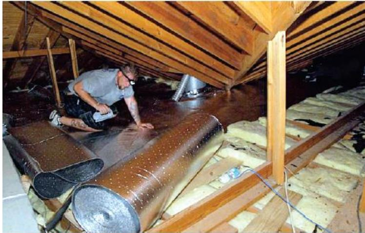
**Figure 1: Arctic Fox Attic Floor Insulation Application (with mass insulation)**
